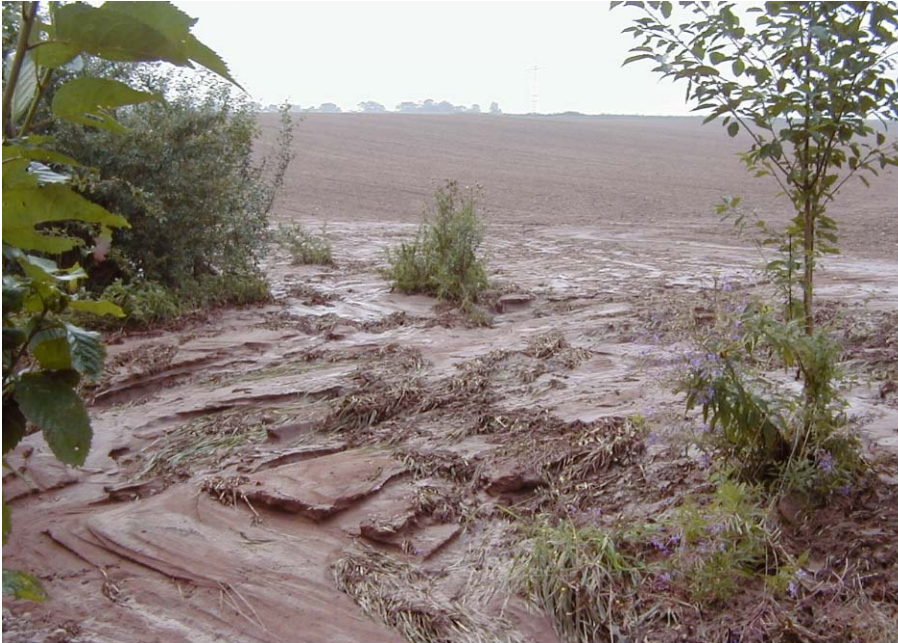
Figure 4: Eroding farmland viewed from Rotbach stream bank
